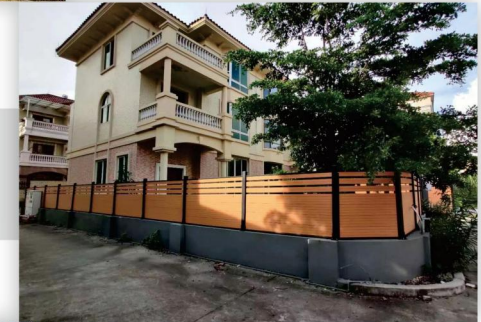
2. Irregular corner fence installation
