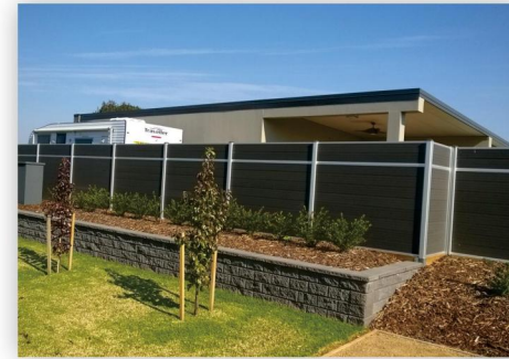
1. Superhigh fence installation
